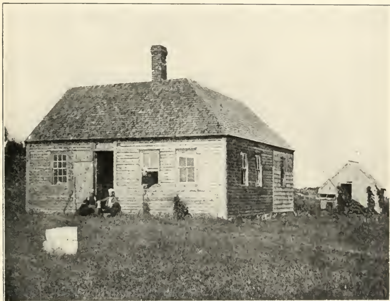
Home of Capt. David Johnson, Bailey's Island, Maine. Built 1788.
